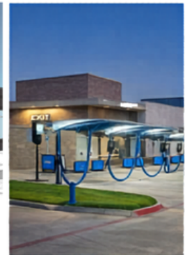
Car Wash Construction
